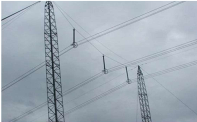
Figure 3 Guyed Cross Rope Suspension
