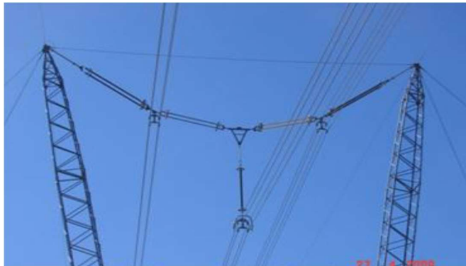
Figure 4 Guyed Cross Rope Suspension Compact
