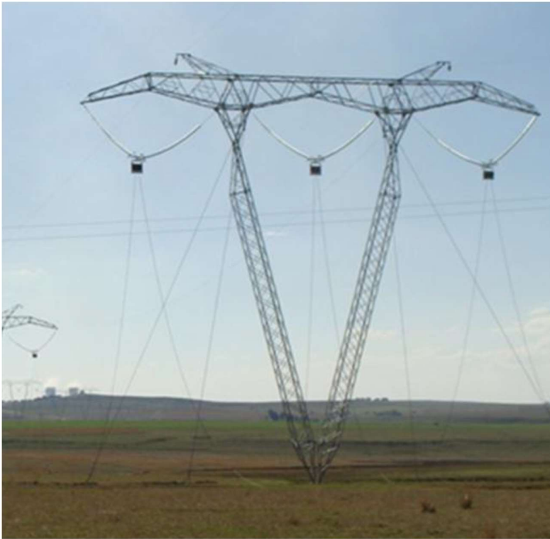
Figure 5 : Guyed V suspension
