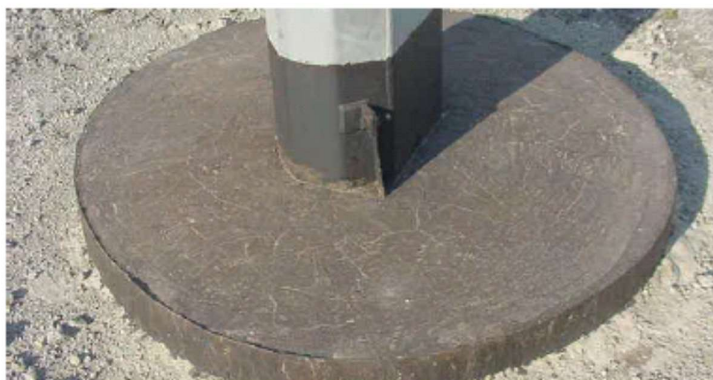
Figure 4-7: Earth-Lug for Additional Earthing on Tubular Steel Structures
